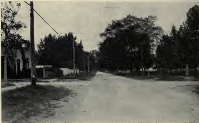
A CONCRETE CROSSROADS WITH CLEAR VISTAS AND WIDE RADIUS CURVES TO REDUCE ACCIDENTS
